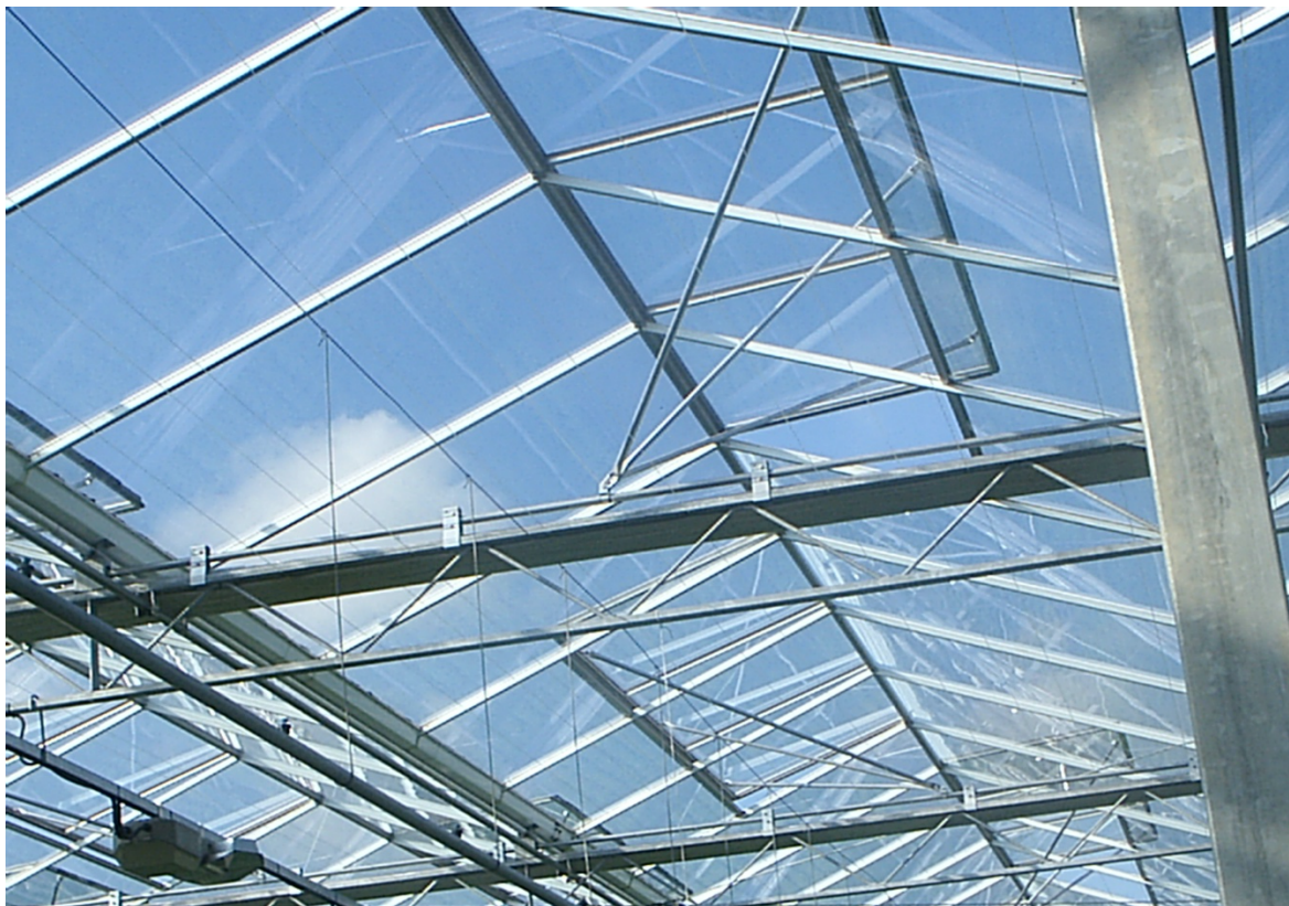
Figure 3 – Greenhouse roof structure type-Venlo (Photo KTBL)
